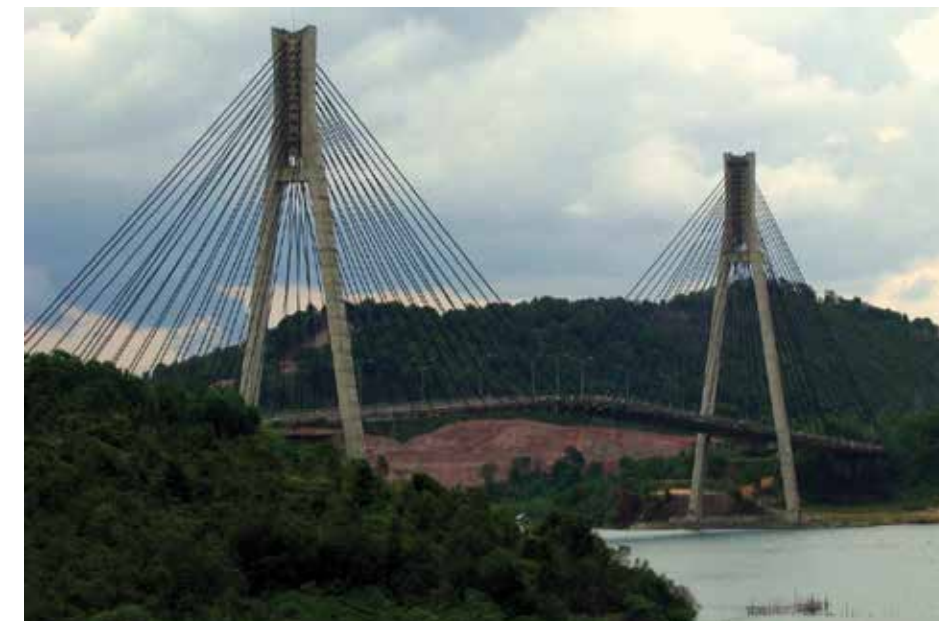
Barelang Bridge, Indonesia. Image: Soham Banerjee.
