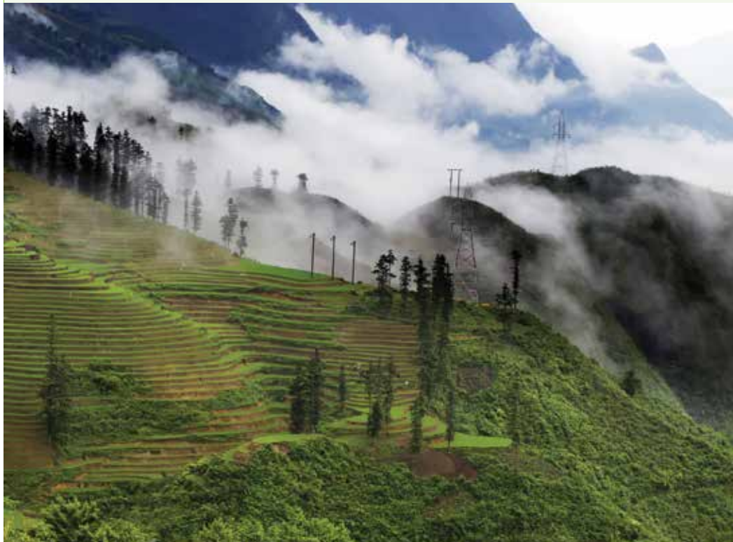
Electricity lines, Vietnam. Image: United Nations.
