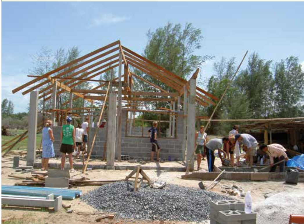
Rebuilding after the tsunami in Thailand. Image: Michael Sarver.
