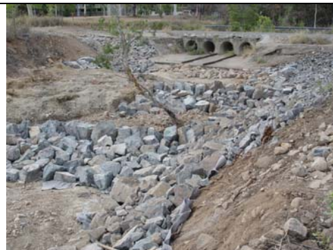
Rock ramp / cascade fishway constructed downstream of culvert to raise water levels in downstream channel – apron fishway under construction (17/12/05)
