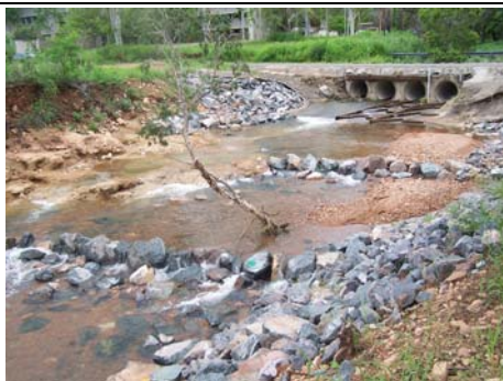
Prototype fishway showing downstream rock ramp cascade – looking U/S (29/01/06)
