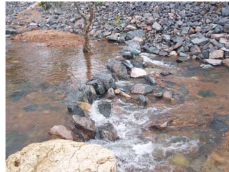
Rock ridge cascade # 2 after January flow – looking from right bank (29/01/06)
