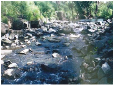
Darebin Creek, Melbourne rock ramp fishway and grade control structure – random rock design (Source: Ross Kapitzke)
