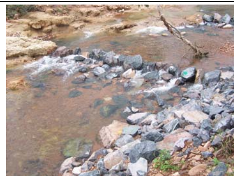
Rock ramp and cascade # 2 –from left bank (29/01/06)
