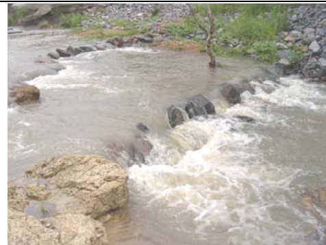
Solander Road rock ramp cascade fishway downstream of pipe culvert / causeway (09/04/06)
