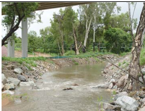
Rock ramp fishway – looking D/S (24/01/05)
