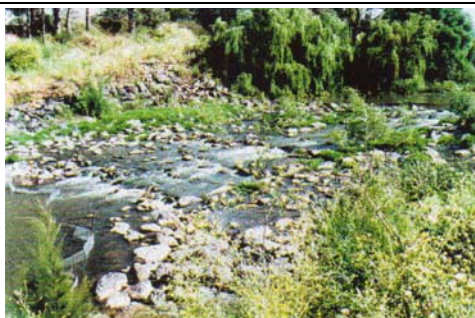
Bell River, NSW rock ramp fishway and grade control structure (Source: Thorncraft and Harris 1997)
