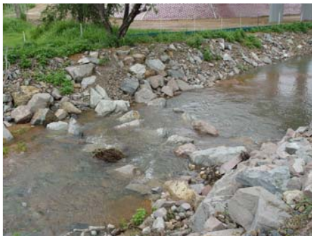
Three rock ridges comprising large boulders with "V" slots between rocks (25/01/05)
