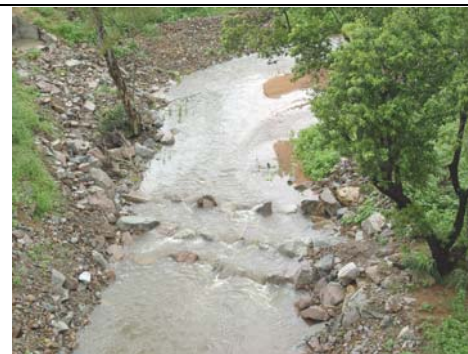
Rock ramp fishway – looking U/S (24/01/05)
