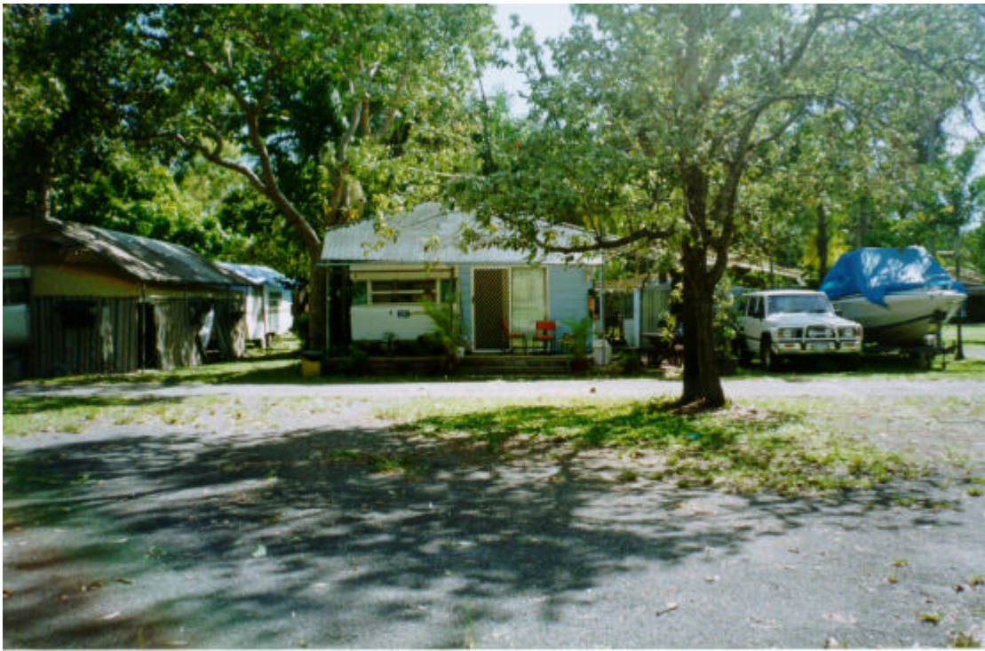
Plate 8. This house structure was built around a caravan (left side of building)
