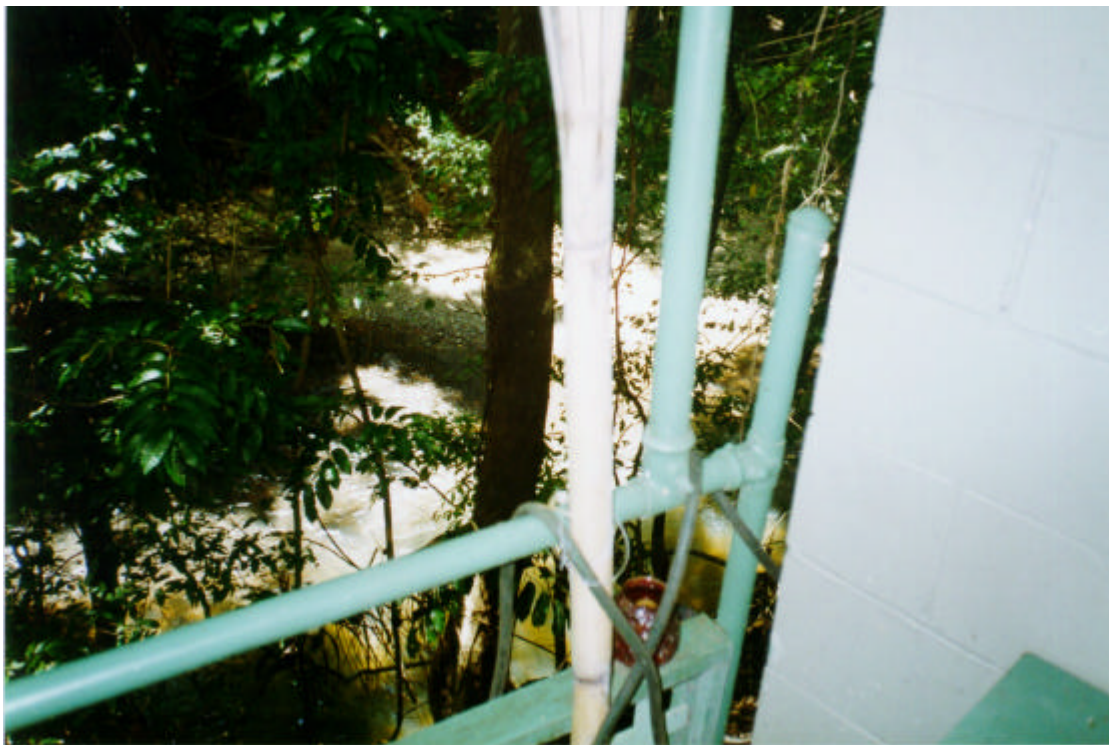
Plate 4. The photo demonstrates a scaffolding and besa-block house structure which was build up around a caravan on the banks of the creek. This structure is highly prone to flooding.
