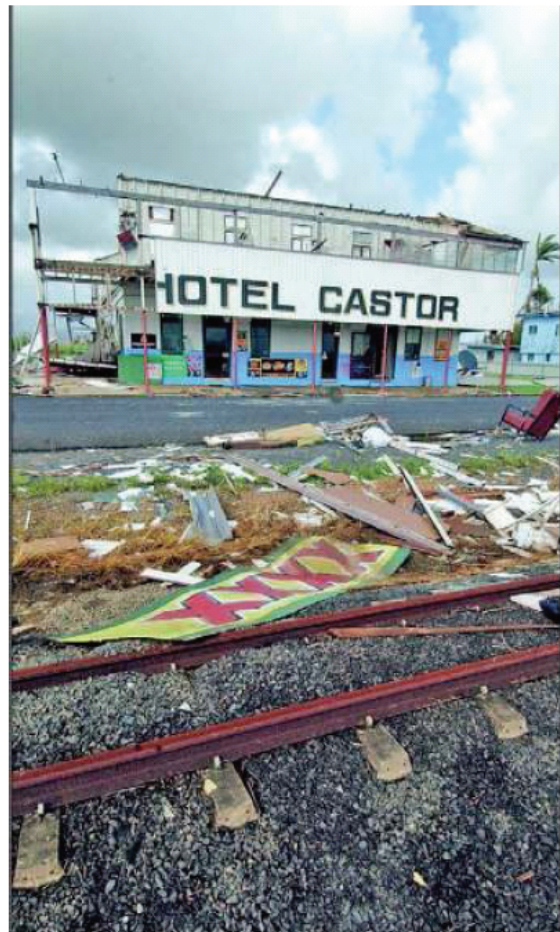
WRECKED ... Mourilyan's Hotel Castor was badly damaged by Cyclone Larry Photo: SCOTT RADFORD-CHISHOLM
