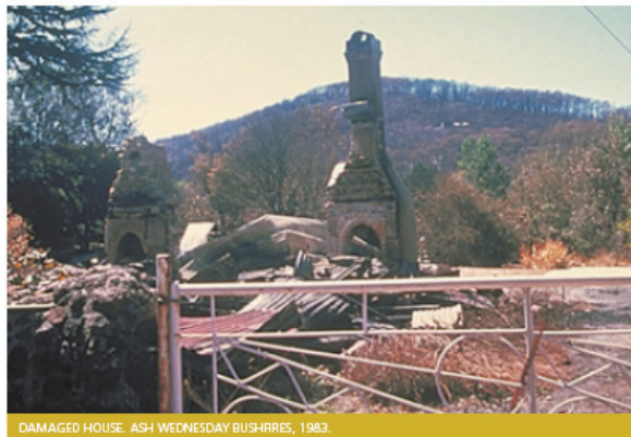
DAMAGED HOUSE. ASH WEDNESDAY BUSH-FIRES, 1983.
