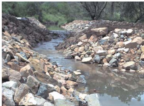
Rock invert crossing in very low flow conditions – looking upstream (02/02/04)
