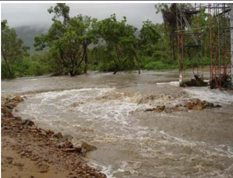
Flow overtopping construction pad – looking upstream (16/01/04)
