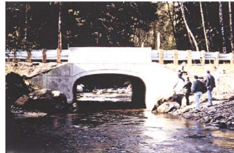
Arch culvert spanning narrow stream channel in north American stream
