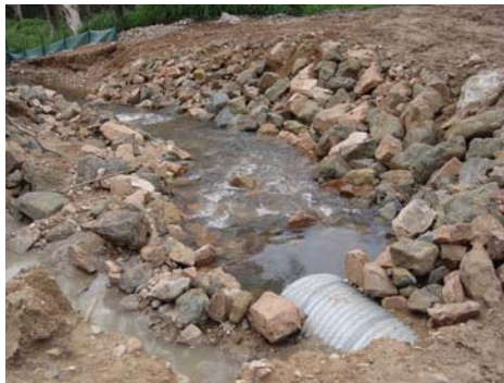
Pipe outlet and downstream diversion drain – looking downstream (14/01/04)
