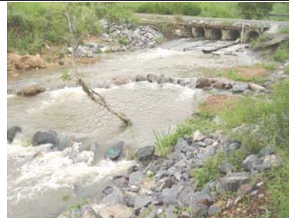
Rock ramp / cascade fishway downstream of culvert structures on Solander Road crossing of University Creek (09/04/06)
