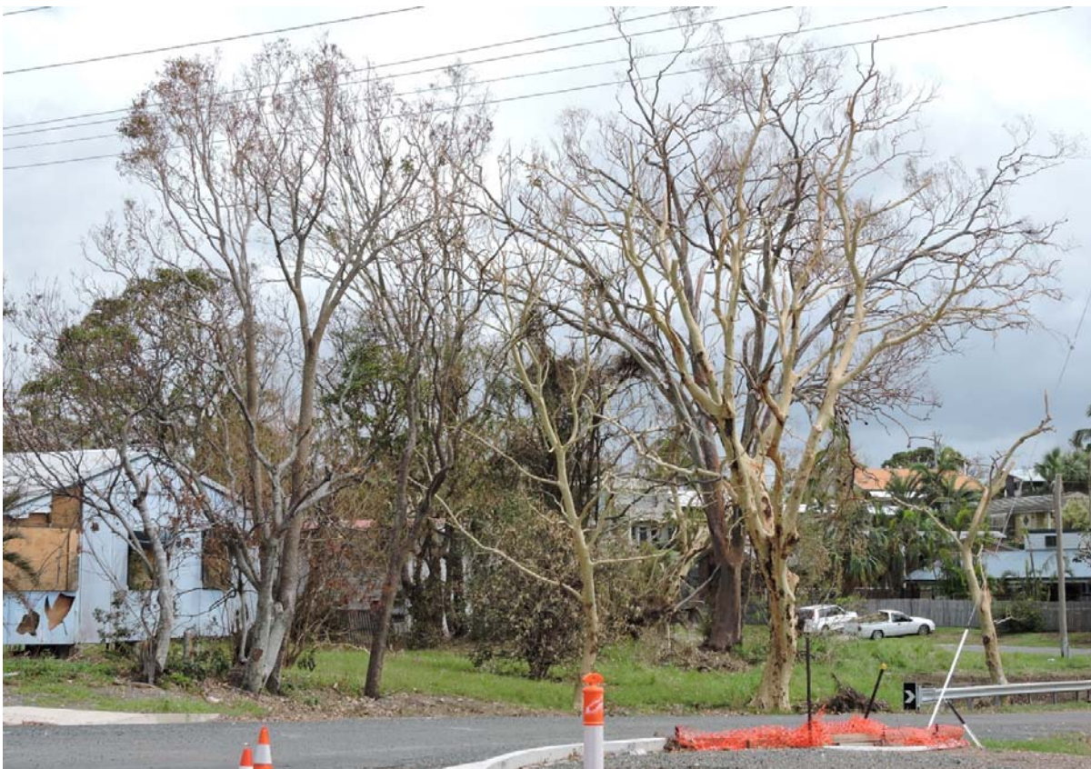
Figure 7. Structural damage and foliage loss, Cannonvale
