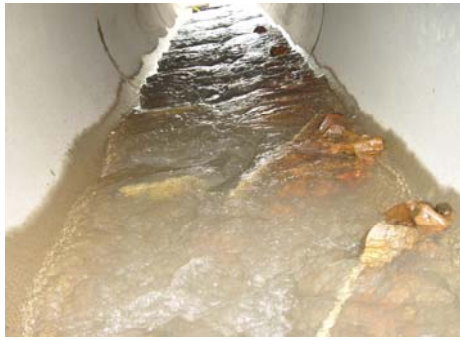
One standard baffle height flow depth – looking D/S (11/04/06)
