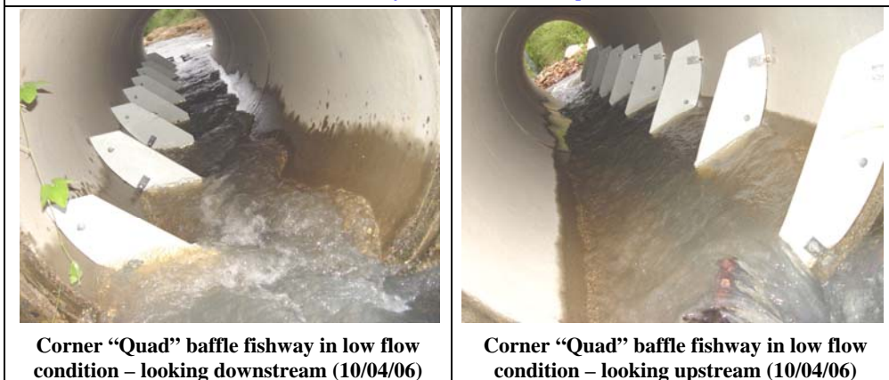
Box G4.1: University Creek Solander Road pipe culvert prototype corner “Quad” baffle fishway (Source: Ross Kapitzke)
