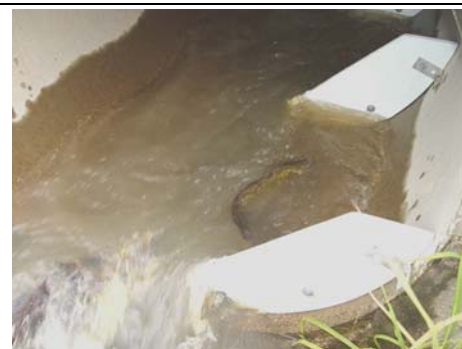
Plotosid catfish resting at D/S end of corner “Quad” baffle fishway – pipe Barrel 2 (09/04/06)
