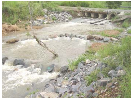
Prototype fishway showing rock ramp and apron baffle fishways – looking U/S (09/04/06)
