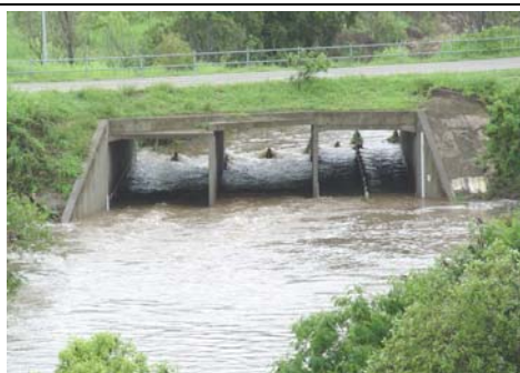
Offset baffle fishway in culvert Barrel 1 – on right looking upstream (16/01/04)
