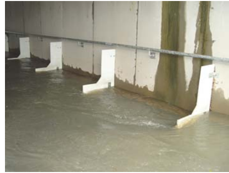
Horizontal leg of baffle emerged, flow depth 250 mm – looking D/S (11/04/06)
