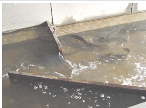
Plotosid catfish moving upstream through offset baffle fishway – resting behind perpendicular baffle (13/01/04)
