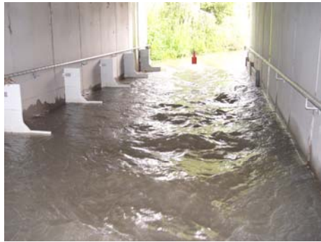
Horizontal leg of baffle emerged, flow depth 250 mm – looking U/S (11/04/06)
