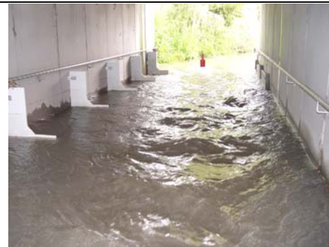
Corner “EL” baffle fishway with flow nearly submerging horizontal leg – looking upstream (-/04/06)
