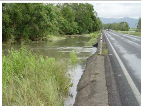
Moderate velocity conditions and no water surface drop at culvert outlet (24/03/06)
