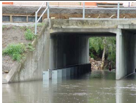
Corner “EL” baffle fishway in culvert Barrel 3 – on left looking upstream (03/02/07)
