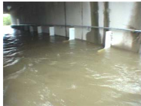
Horizontal leg of baffle just submerged, flow depth 350 mm – looking D/S (27/01/06)
