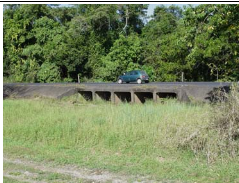
Box culvert installed in low gradient waterway on floodplain (29/09/05)
