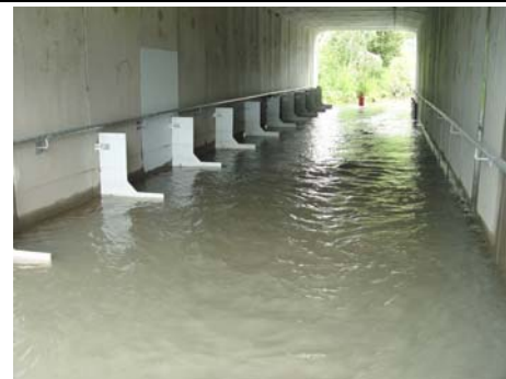
Corner “EL” baffle fishway in low flow condition – looking upstream (10/04/06)
